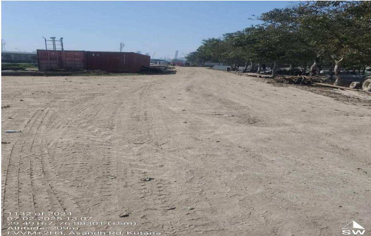
Photograph 1: Inadequate arrangements for dust suppression within the premises.
